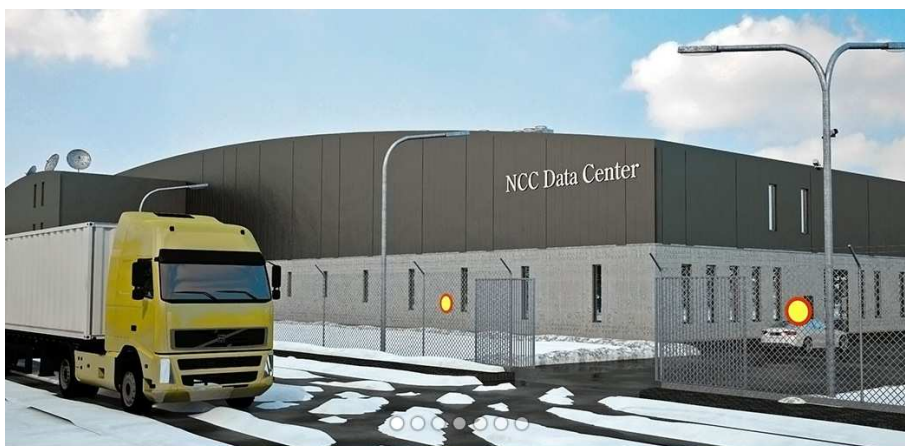
Figur 2-15: NCC Data Center. Kilde: NCC: NCC – Data Center - Scharc
