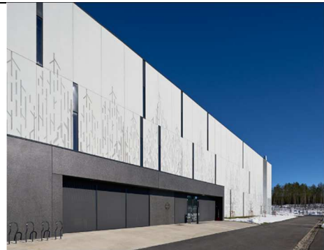
Figur 2-8: Datasenter i Fetsund. Kilde: Norway Data Center Co-location Services In Oslo Fetsund | DigiPlex
