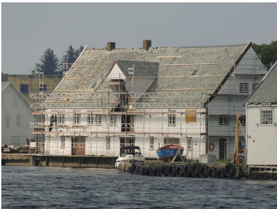
Bergesenhuset under restaurering.
